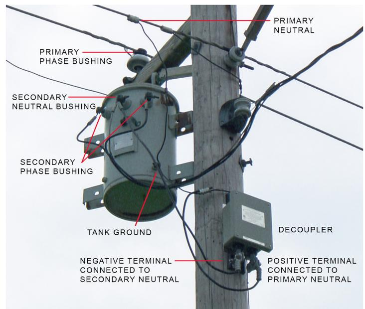
Figure 6. Decoupler installation at a single-phase pole-mounted transformer.
