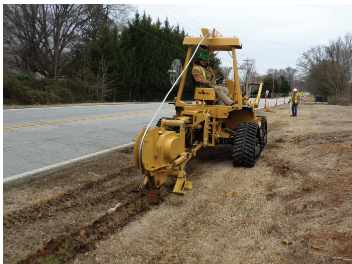
Figure 4: Plowing application of linear zinc mitigation system
