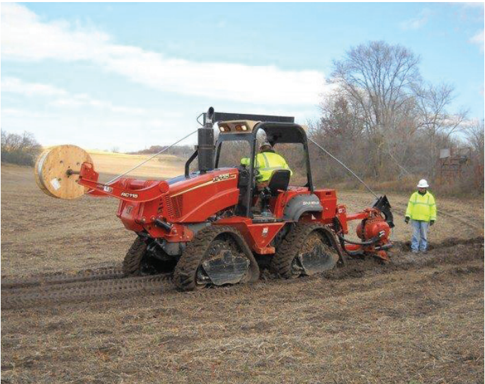
Figure 2: Typical installation of zinc mitigation system
