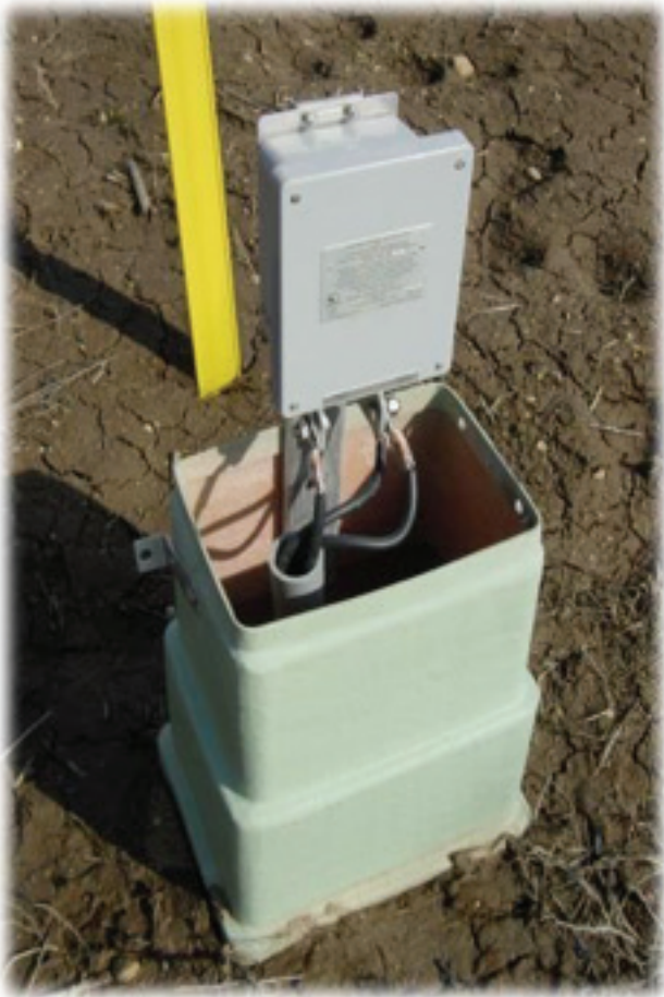
Figure 3: Dairyland PCR in MTP-36 pedestal (with cover removed) on AC mitigation project along high voltage AC right-of-way
