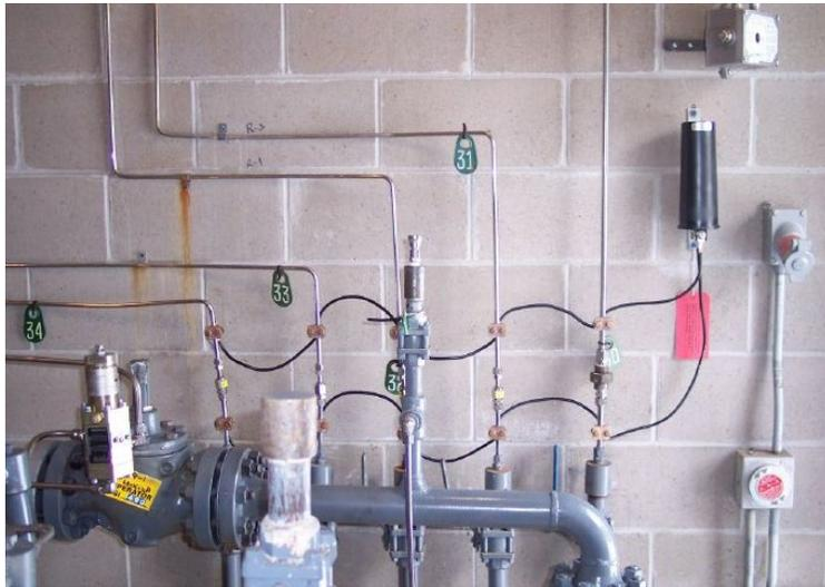
Figure 15: Multiple isolated fittings protected by decoupler
